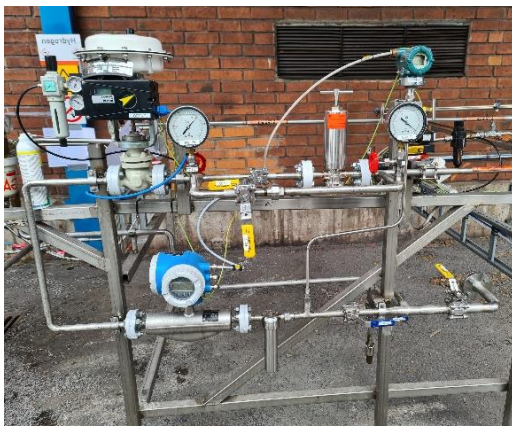
Figure 7. New control systems were installed for hydrogen (left) and nitrogen (right).
