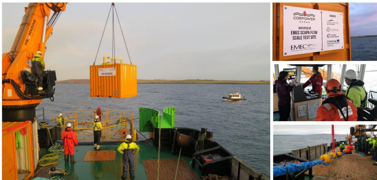
Figure 6. Microgrid contained installation and 300m cable lay between WEC and Microgrid.
