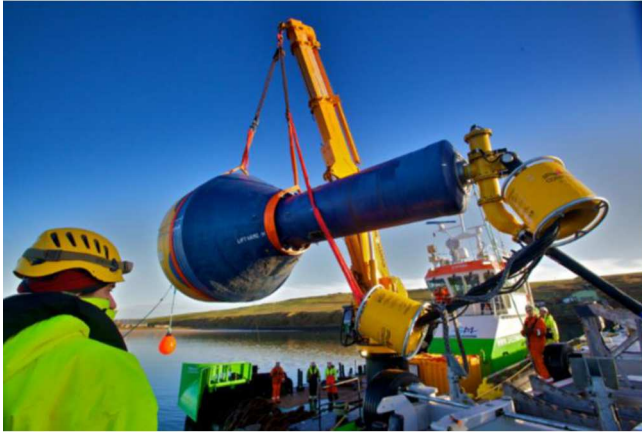
A. WEC lift into water by the multicat's on-board crane
