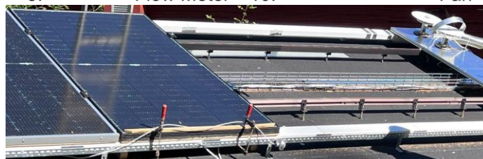
Fig. 1: Open-to-ambient setup with listed sensors and photo of the installation.
