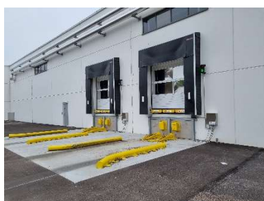
Loading gates at Bjelin factory in Viken
