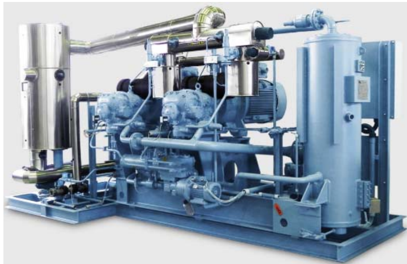
Figure 4-5 Typical standard chiller unit (Source: XXXX)
