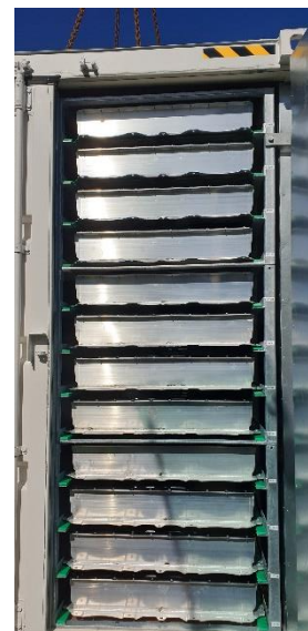
Figur 2. Batteripack staplade i rack.
